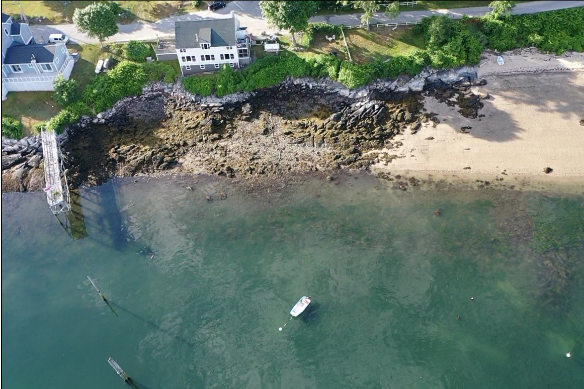
Photograph Three. Additional overview of project site. Photographer: Tim Forrester, Atlantic Environmental, LLC Date: June 29, 2022.
